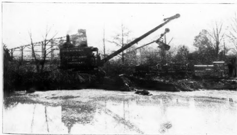
Excavating Material at Grovemont
